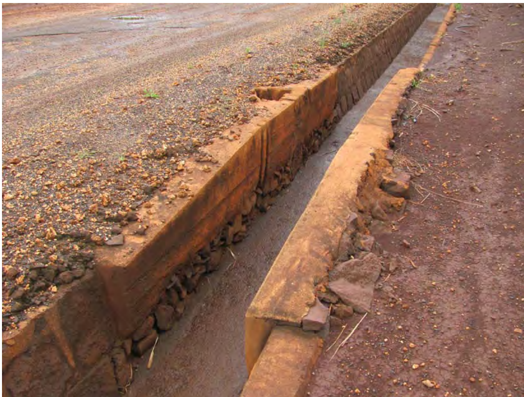
Figure 52. Site 7159 Section 2 fourth sluice gate complex, view to the south.
