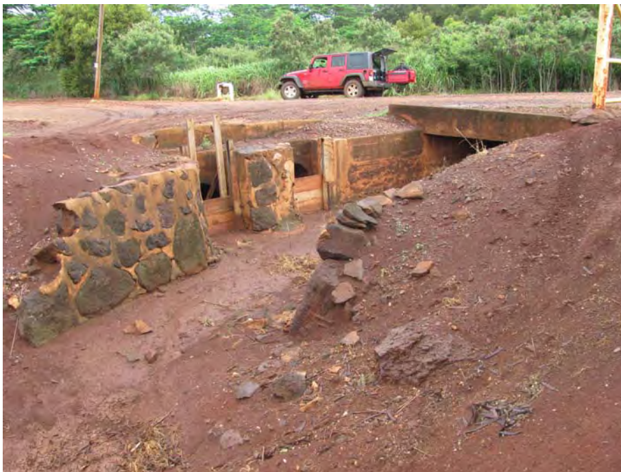
Figure 46. Site 7159 Section 1 sluice gate complex, view to the southwest.
