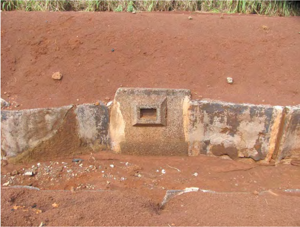
Figure 110. Site 7169 Section 2 sluice gate, view to west.
