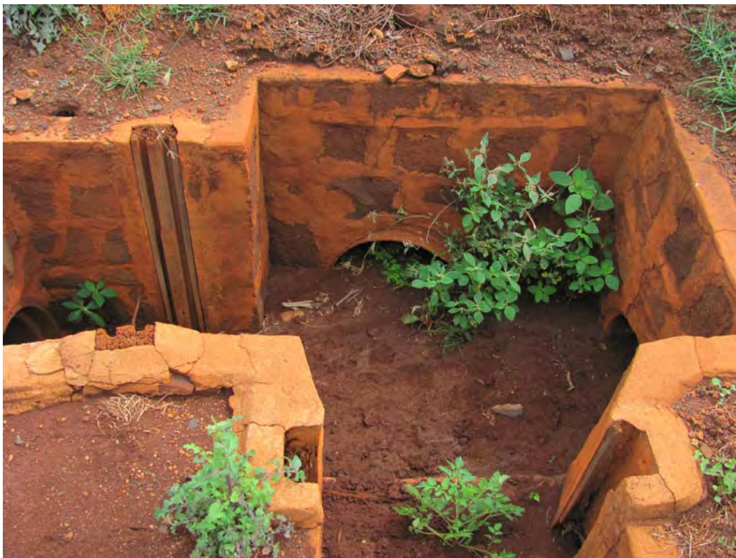
Figure 79. Site 7159 Section 12 sluice gate complex, view to the north.
