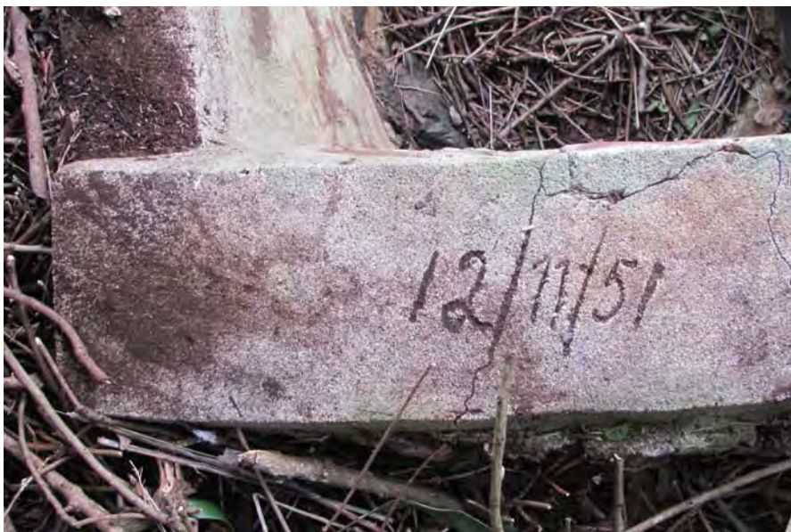
Figure 105. Site 7169 Section 1 date incised into the cement above the pipe, overview.
