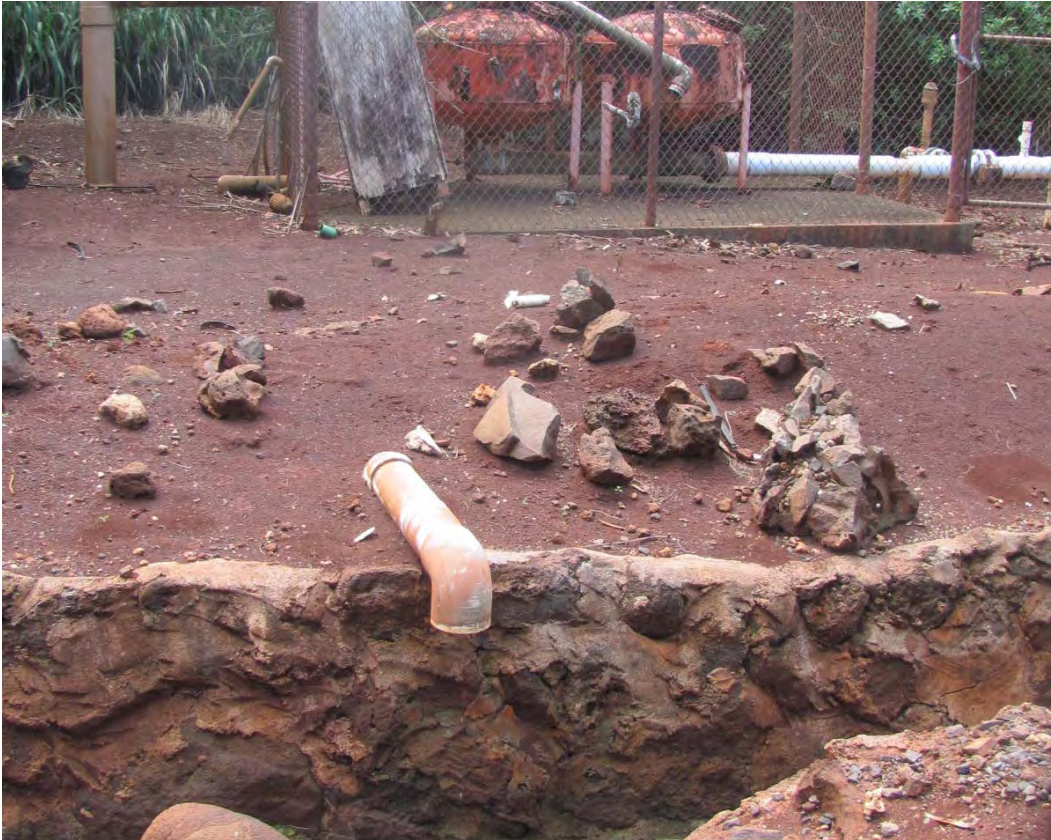
Figure 131. Site 7170 Section 9 PVC pipe and nearby pressure tanks, view to the south.
