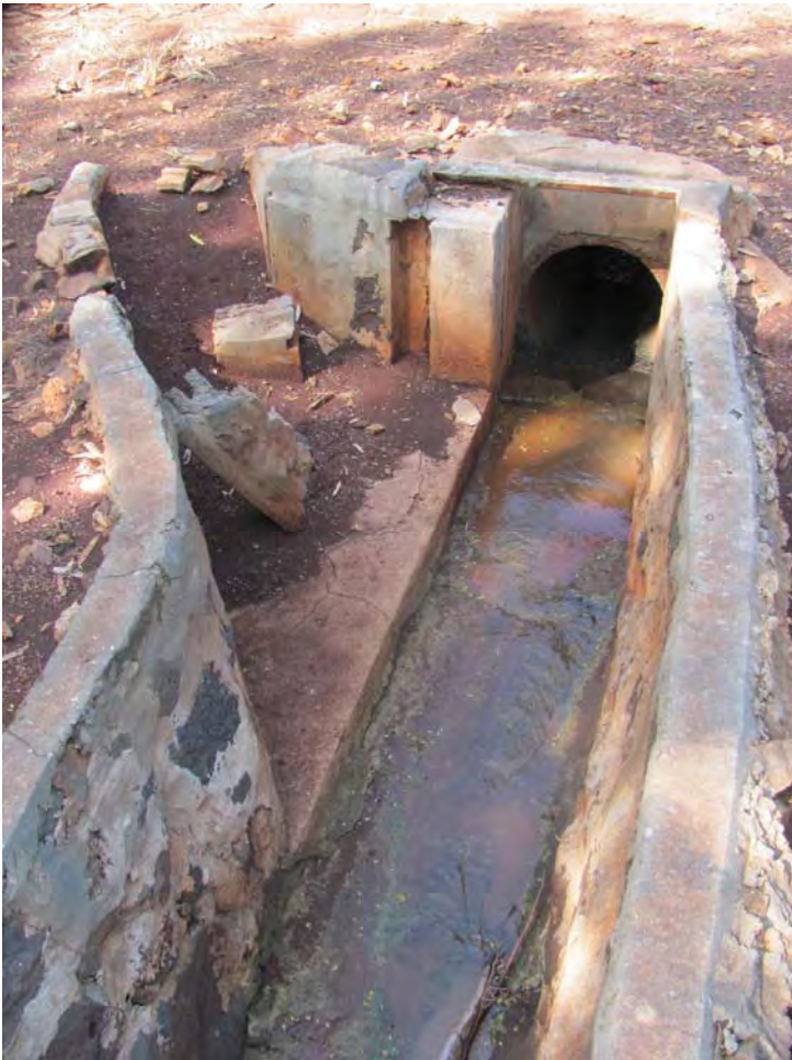
Figure 123. Site 7170 Section 4 makai end, view to the west.
