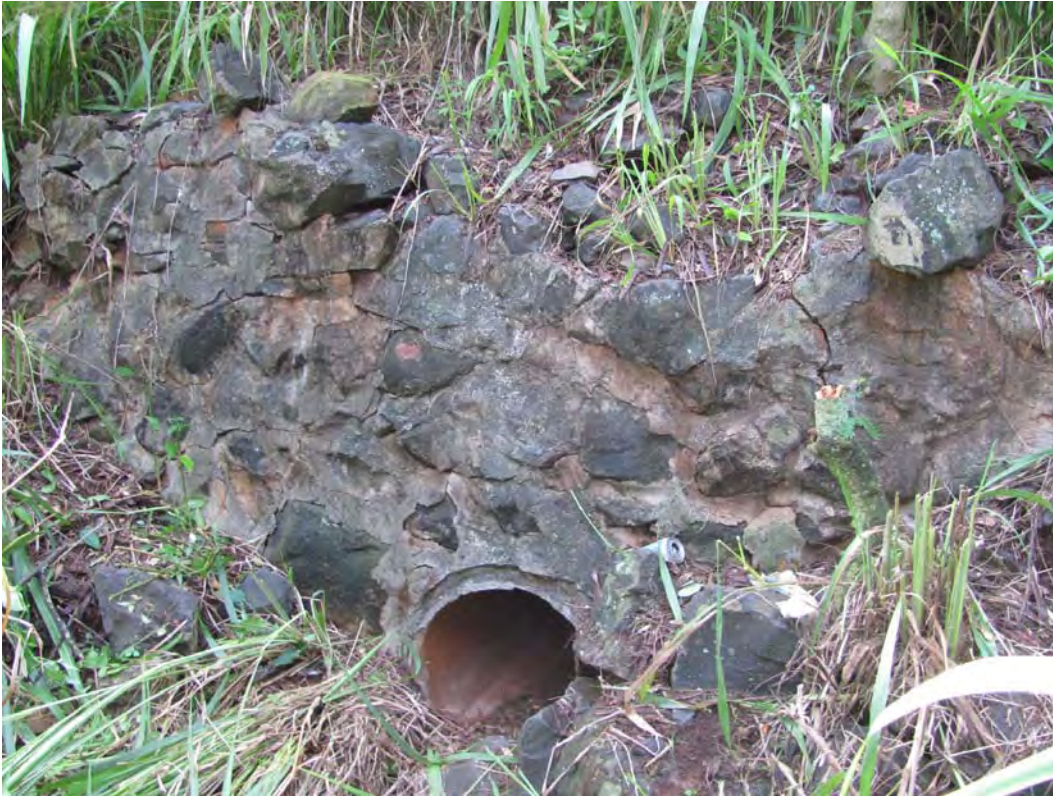
Figure 94. Site 7165 makai revetment, view to the southeast.
