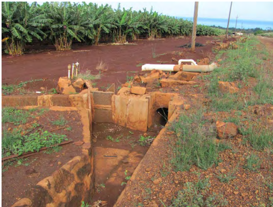
Figure 75. Site 7159 Section 11 first sluice gate complex, view to the south.
