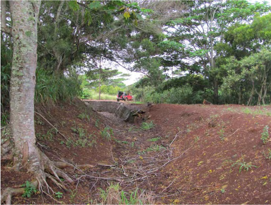
Figure 47. Site 7159 Section 1 northern portion of main ditch, view to the south.
