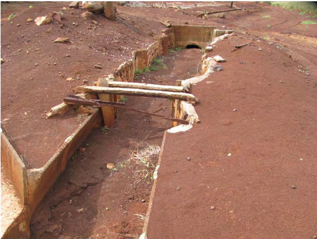
Figure 107. Site 7169 Section 1 sluice complex at Mid-Line Road, view to the south.
