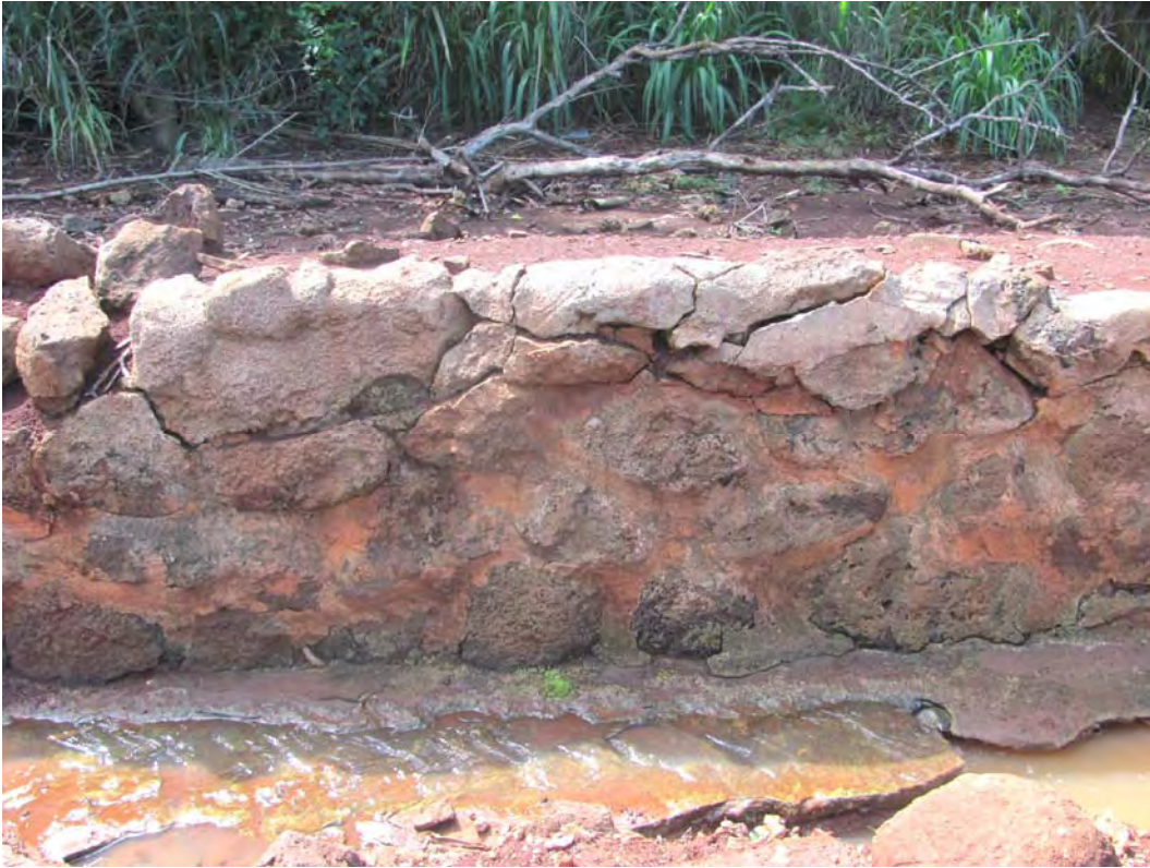
Figure 126. Site 7170 Section 6 intact south wall, view to the south.
