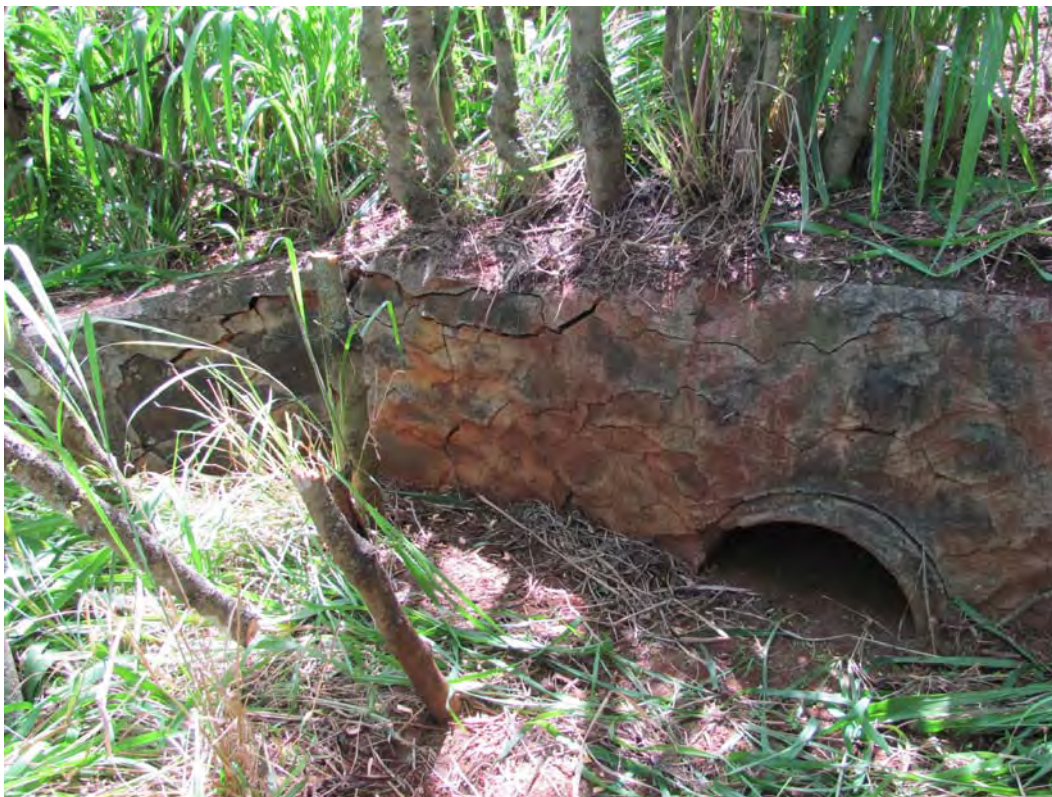
Figure 96. Site 7166 makai revetment, view to the east.
