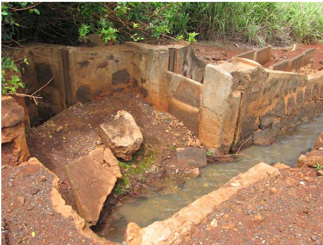
Figure 59. Site 7159 Section 6 sluice gate complex, view to the south.
