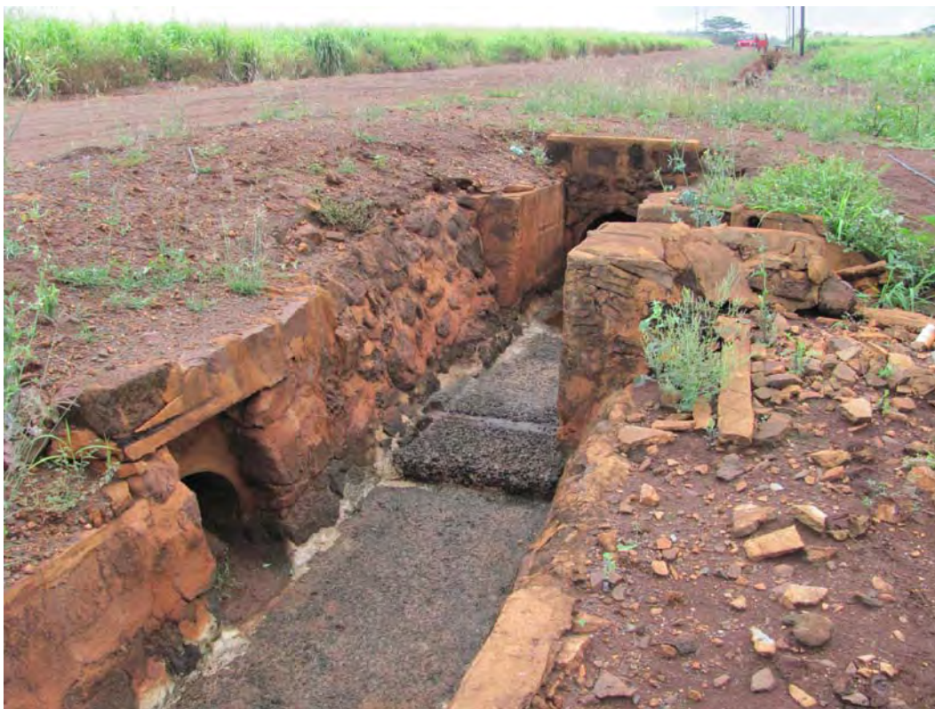
Figure 68. Site 7159 Section 10 first sluice gate complex, view to the north.
