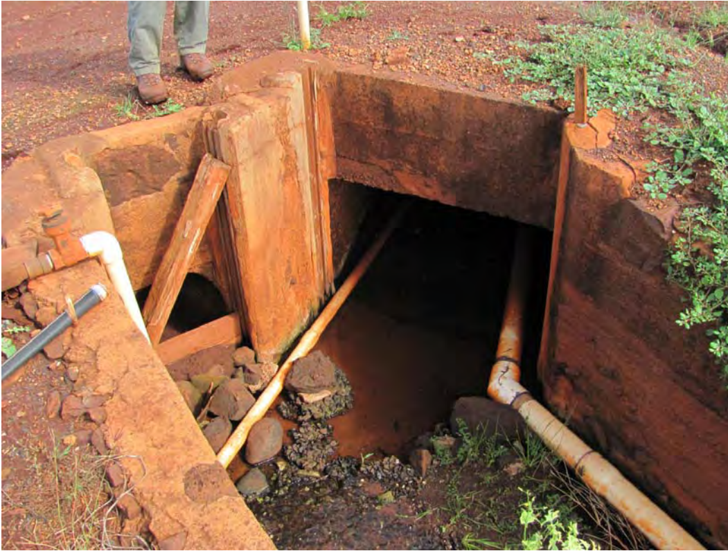
Figure 73. Site 7159 Section 10 fifth sluice gate complex, view to the southwest.
