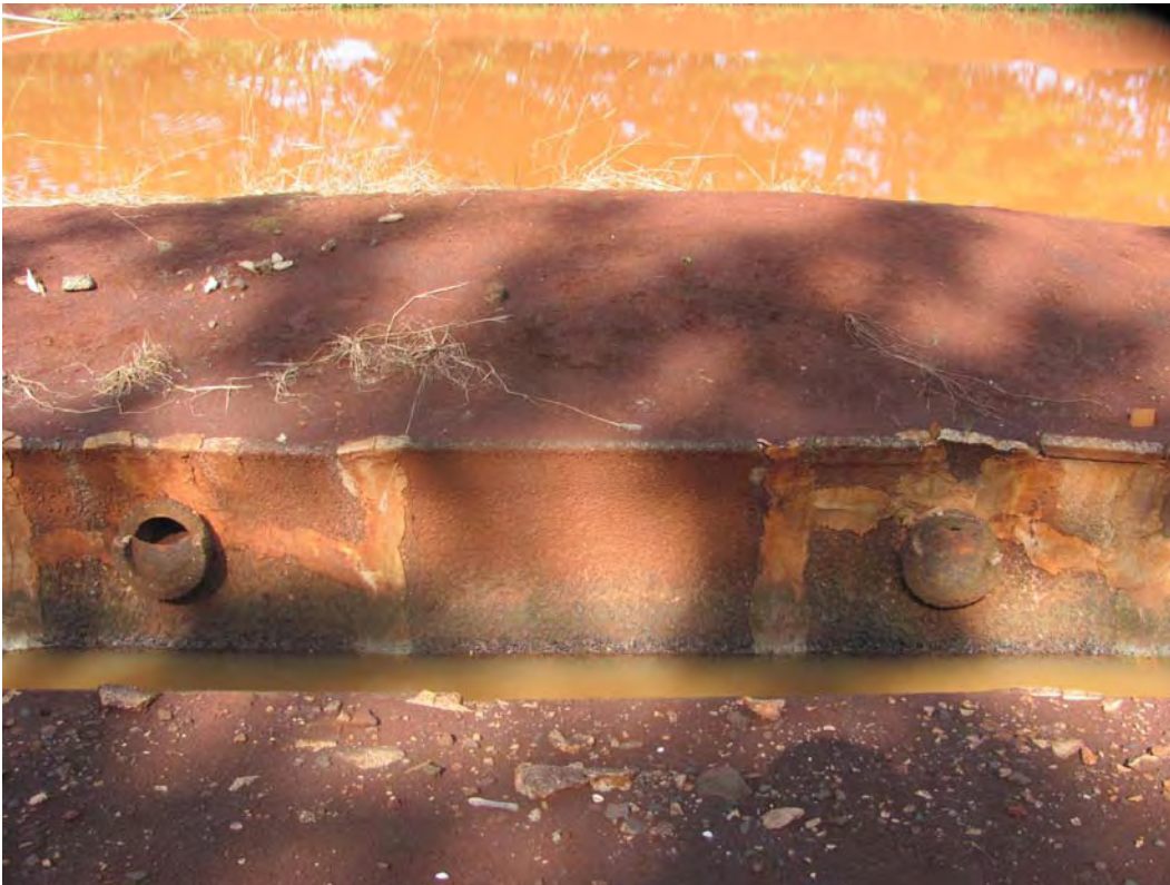
Figure 118. Site 7170 Section 2 concrete overflow pipes, view to the west.
