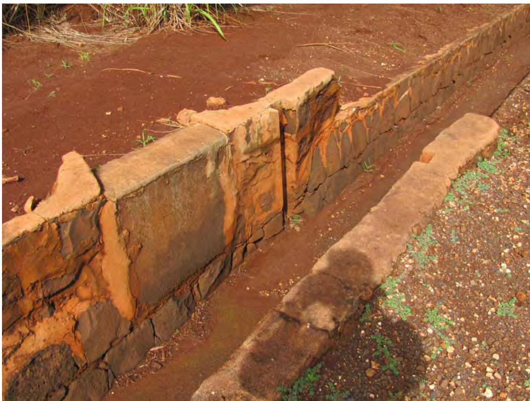
Figure 49. Site 7159 Section 2 first sluice gate complex, view to the south.
