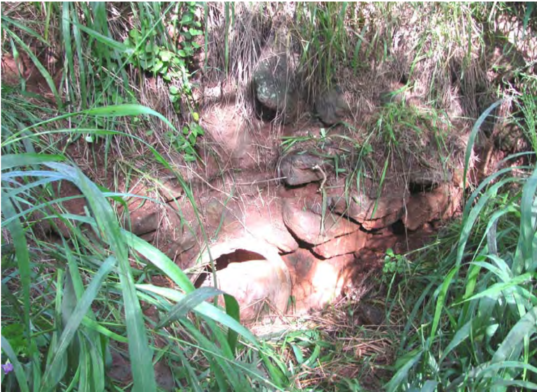
Figure 97. Site 7167 mauka revetment, view to the west.
