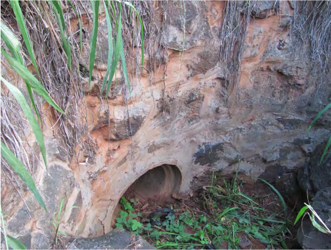
Figure 88. Site 7163 mauka revetment, view to the west.
