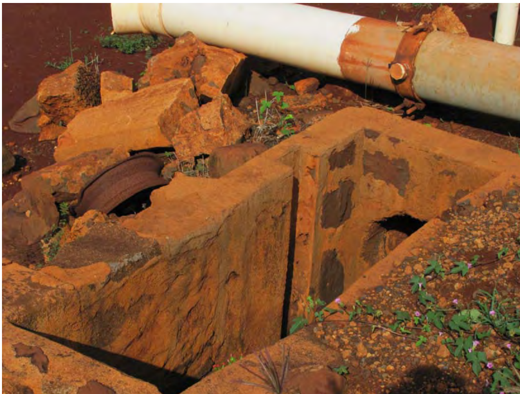
Figure 76. Site 7159 Section 11 second sluice gate, view to the south.
