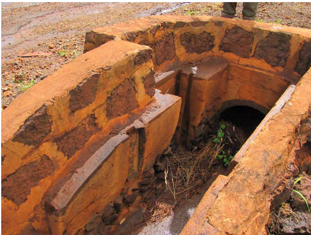
Figure 53. Site 7159 Section 3 sluice gate complex, view to the south.
