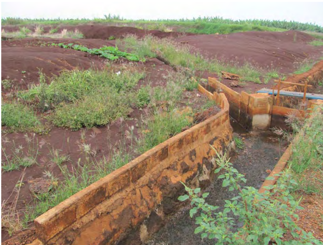
Figure 71. Site 7159 Section 10 third sluice gate complex, view to the south.
