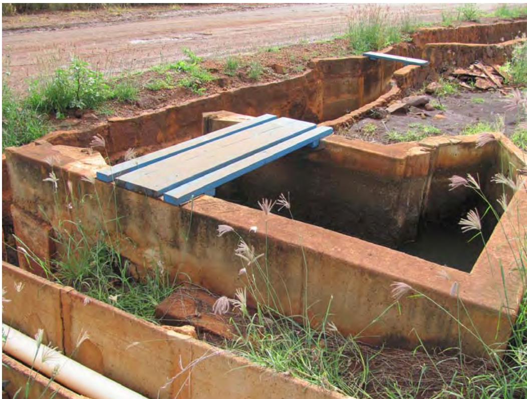
Figure 72. Site 7159 Section 10 fourth sluice gate complex, view to the north.
