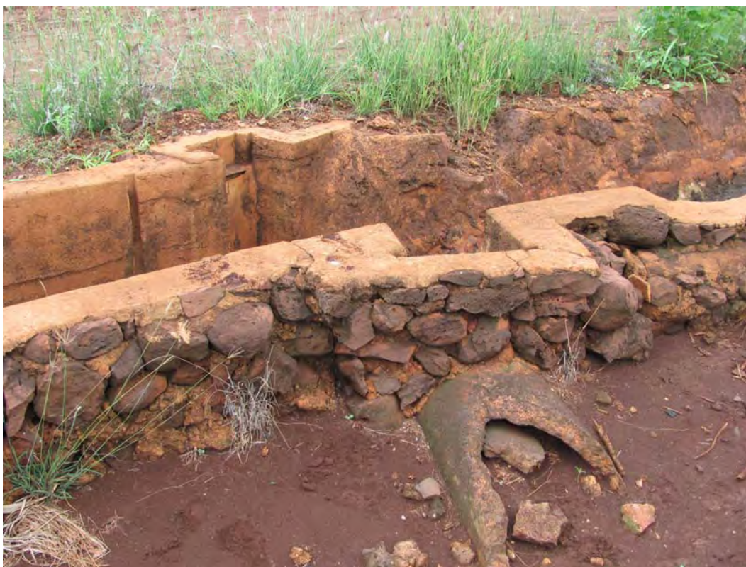
Figure 69. Site 7159 Section 10 second sluice gate complex, view to the south.
