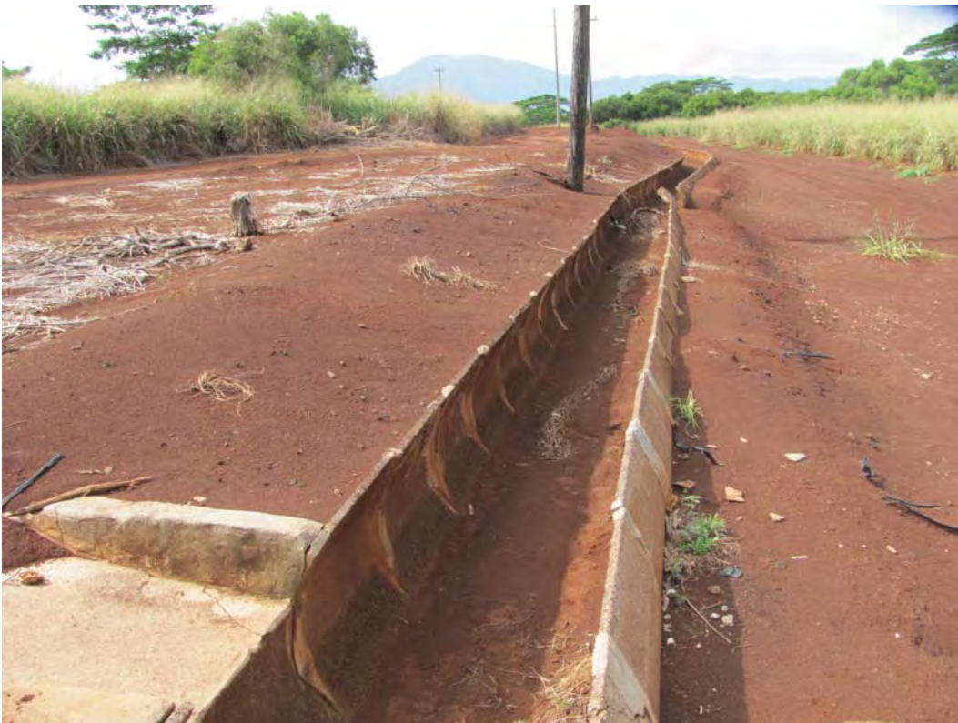
Figure 109. Site 7169 Section 2, view to southwest.
