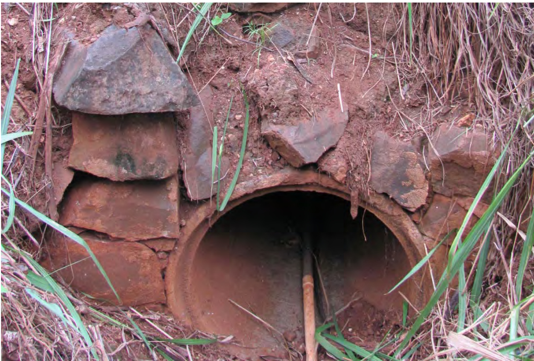
Figure 95. Site 7166 mauka revetment, view to the west.
