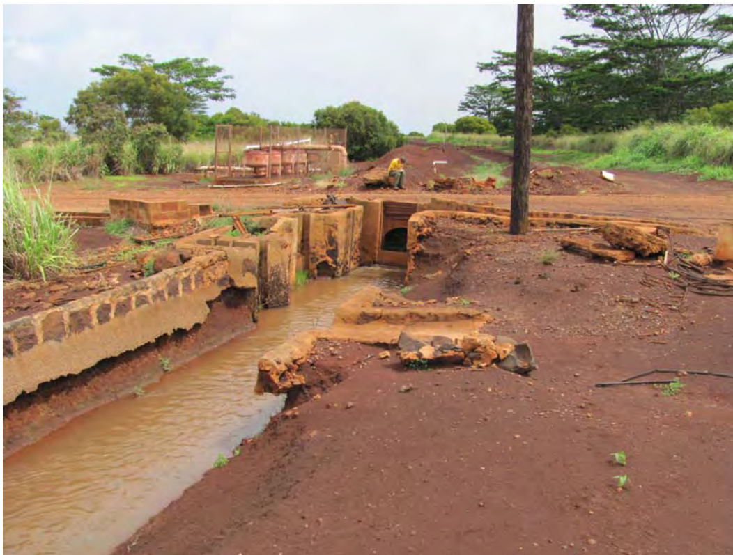
Figure 55. Site 7159 Section 4 sluice gate complex, view to north.
