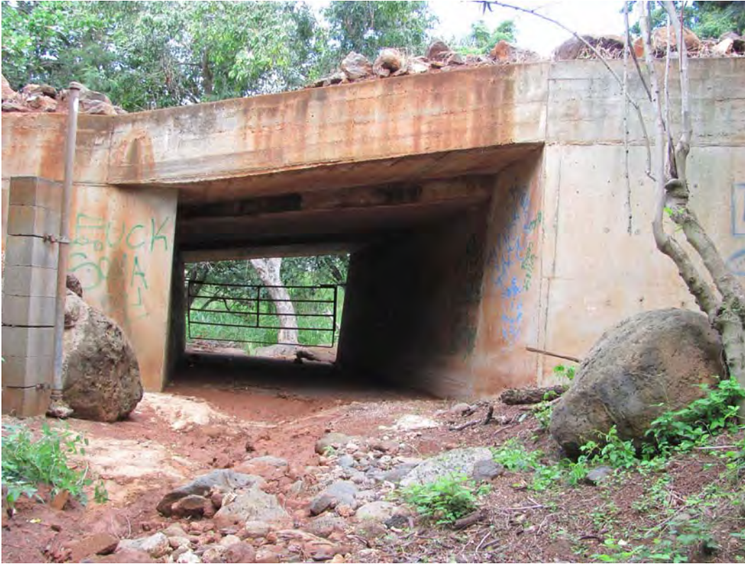
Figure 101. Site 7167 mauka edge, view to the north.
