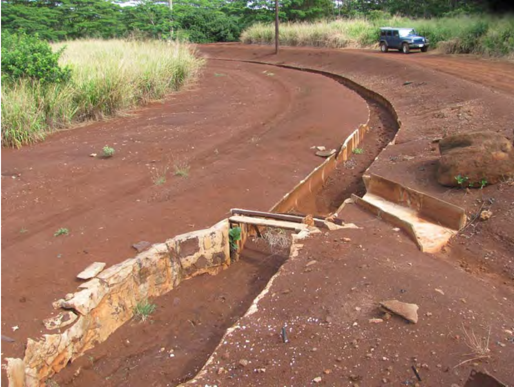
Figure 106. Site 7169 Section 1 surface drainage channel, view to the north.
