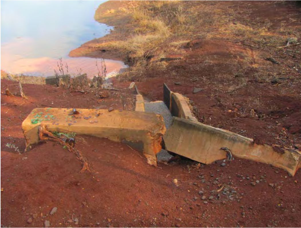
Figure 113. Site 7170 Section 1 outlet to reservoir, view to the northeast.
