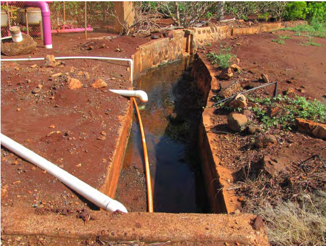
Figure 74. Site 7159 Section 11 north of Kawaihoa Road, view to the north.
