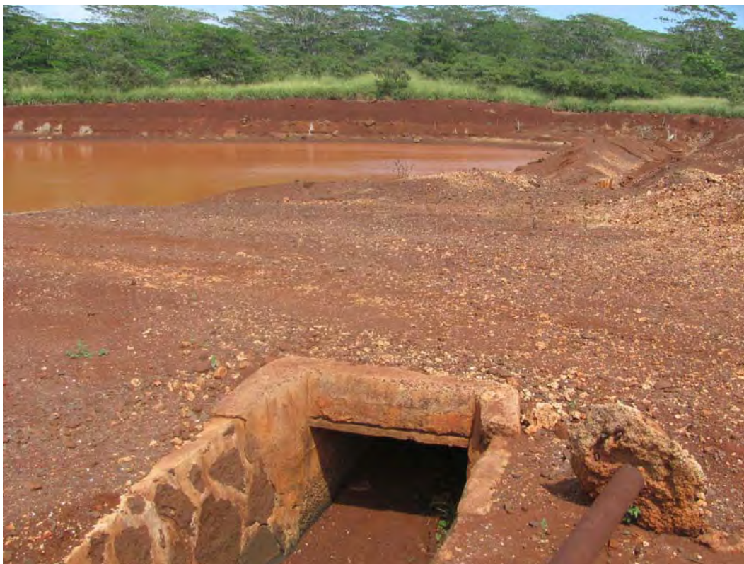
Figure 142. Site 7170 Section 14 northeast end and reservoir beyond, view to the northeast.
