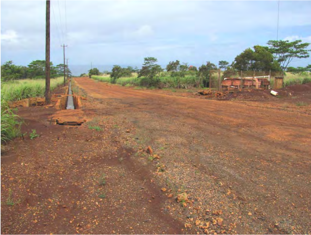
Figure 19. Kawaiiloa Road Corridor, middle section, view to the west.
