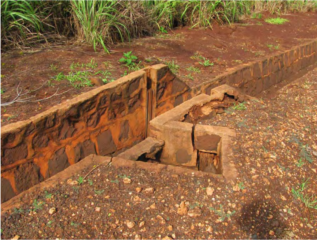
Figure 50. Site 7159 Section 2 second sluice gate complex, view to the south.
