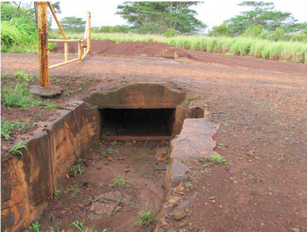
Figure 48. Site 7159 Section 1 north side sluice gate complex, view to the south.
