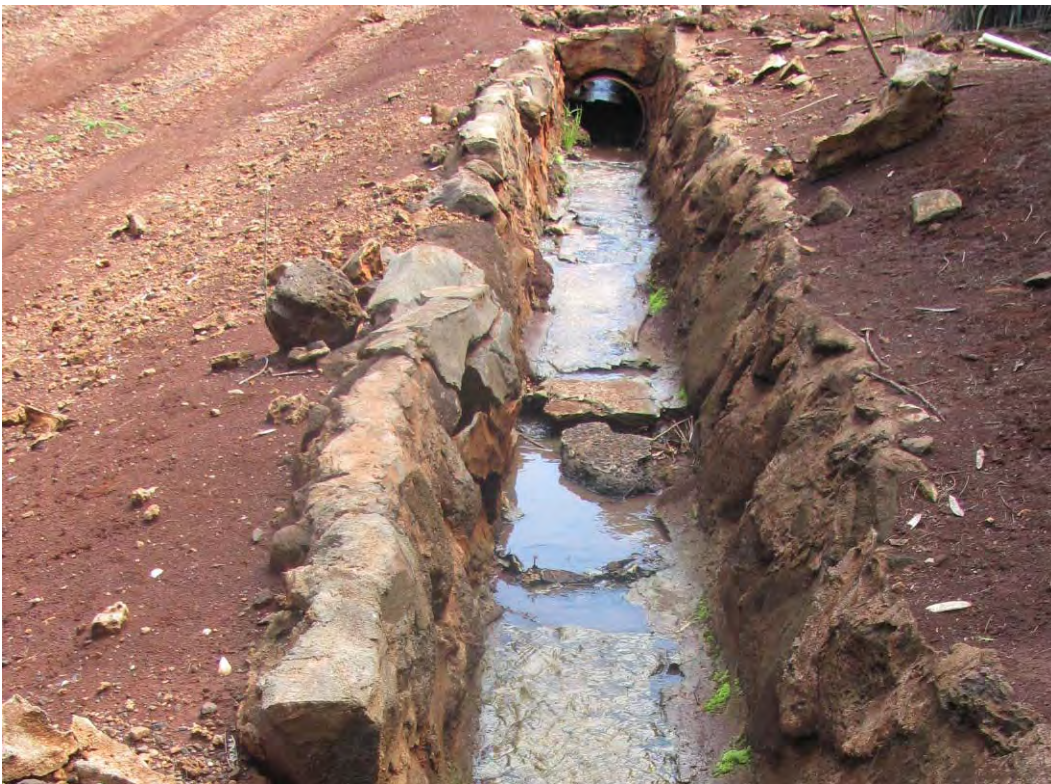
Figure 132. Site 7170 Section 10 mauka end, view to the east.
