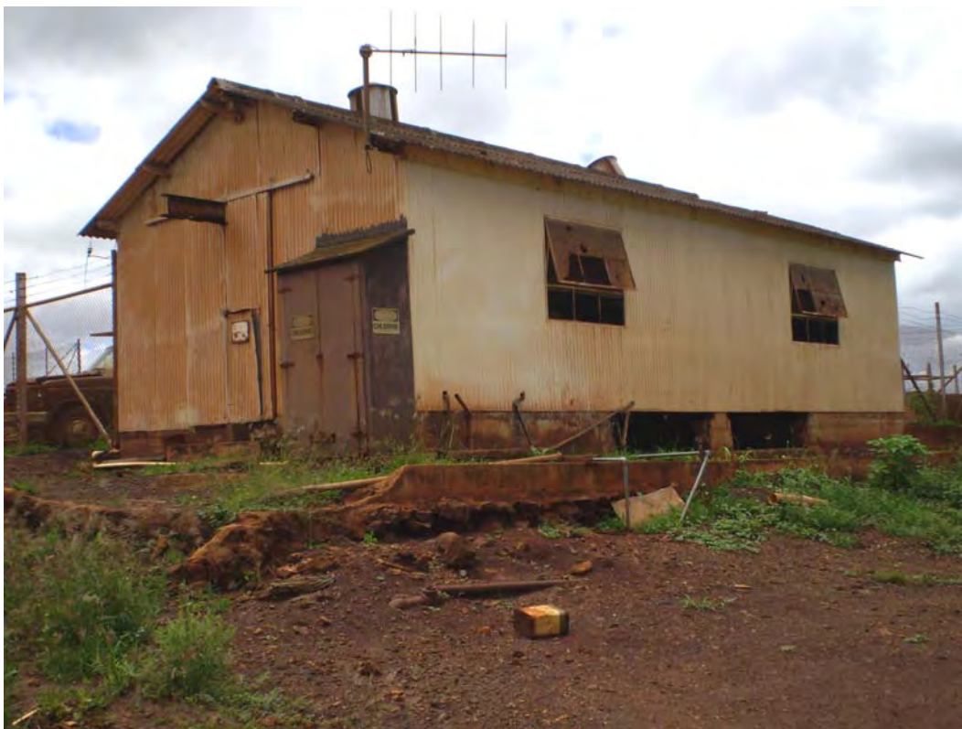
Figure 80. Site 7159 Section 14 building, view to the northeast.
