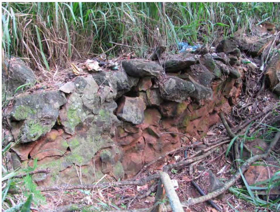
Figure 93. Site 7165 mauka revetment, view to the northwest.
