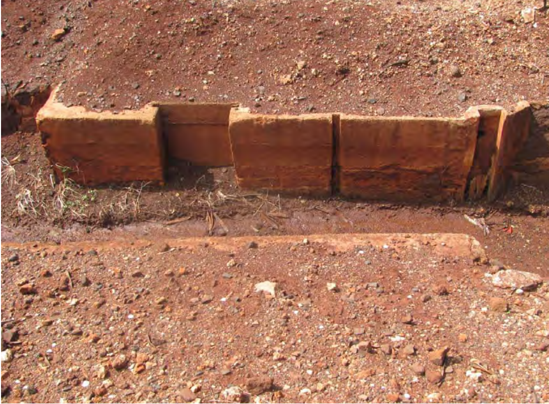
Figure 140. Site 7170 Section 14 sluice complex in the west wall, view to the west.
