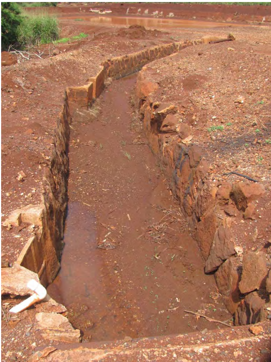
Figure 139. Site 7170 Section 14, view to the north.
