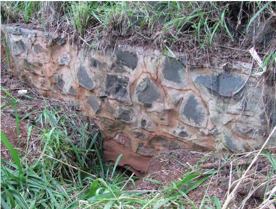
Figure 89. Site 7163 makai revetment, view to the east.
