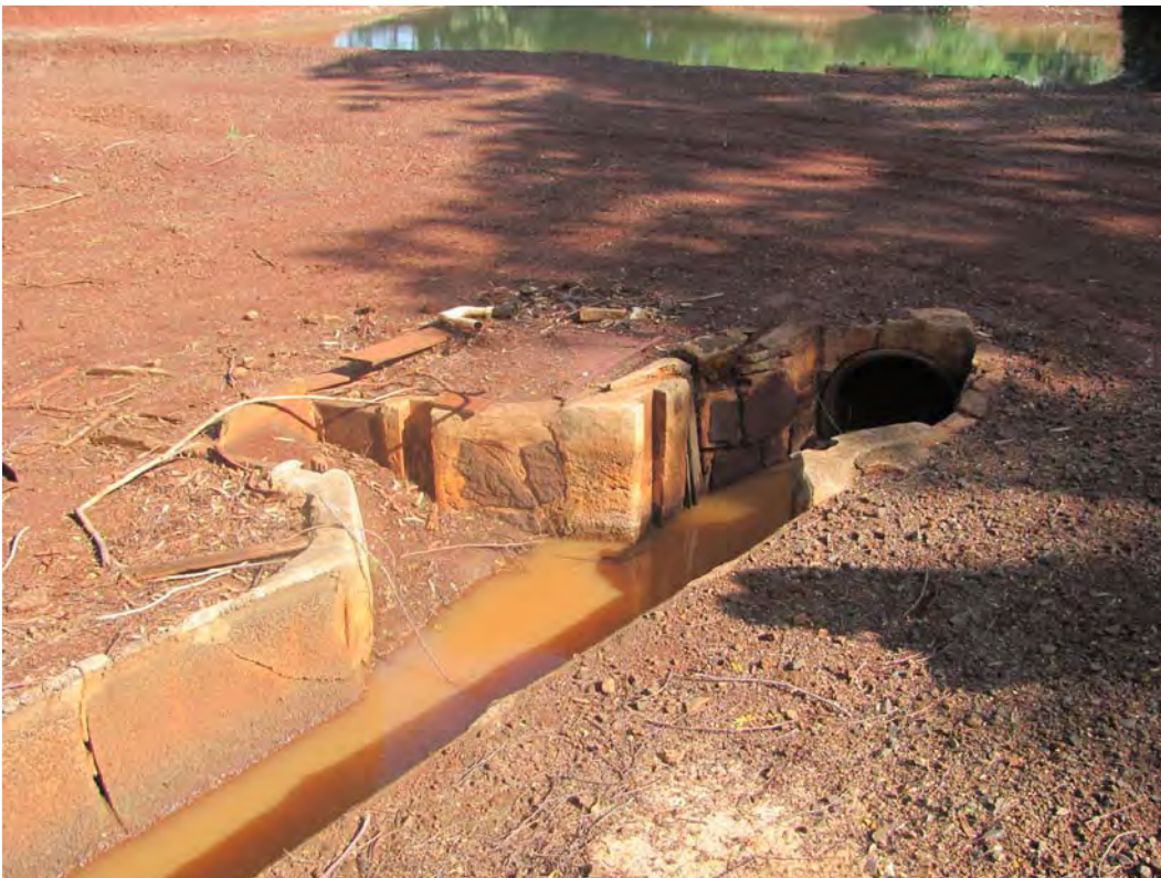
Figure 114. Site 7170 Section 1 sluice complex at north end, view to the north.
