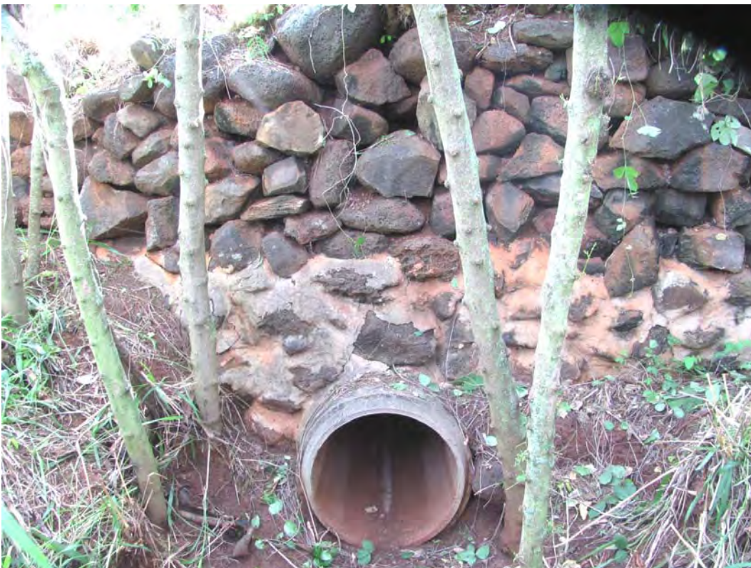
Figure 98. Site 7167 makai revetment, view to the east.
