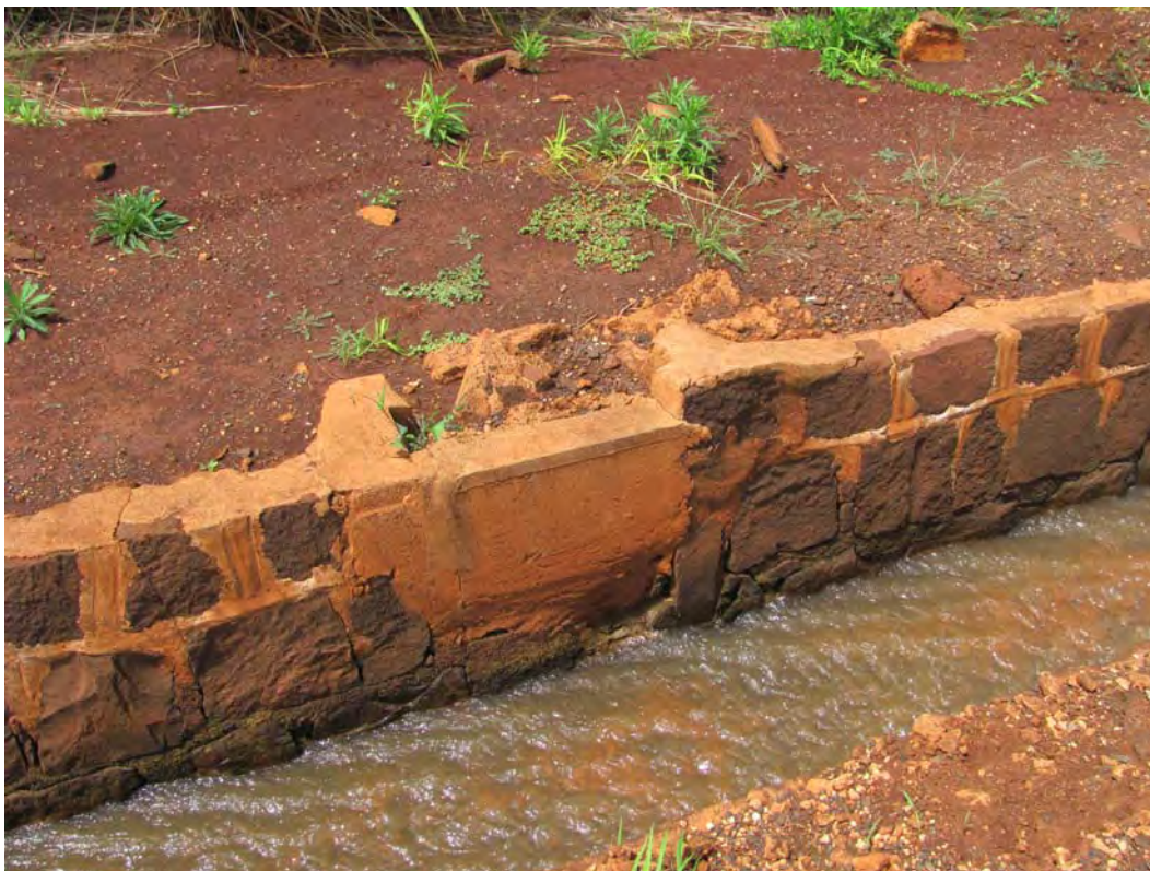
Figure 56. Site 7159 Section 4 blocked side sluice, view to the south.
