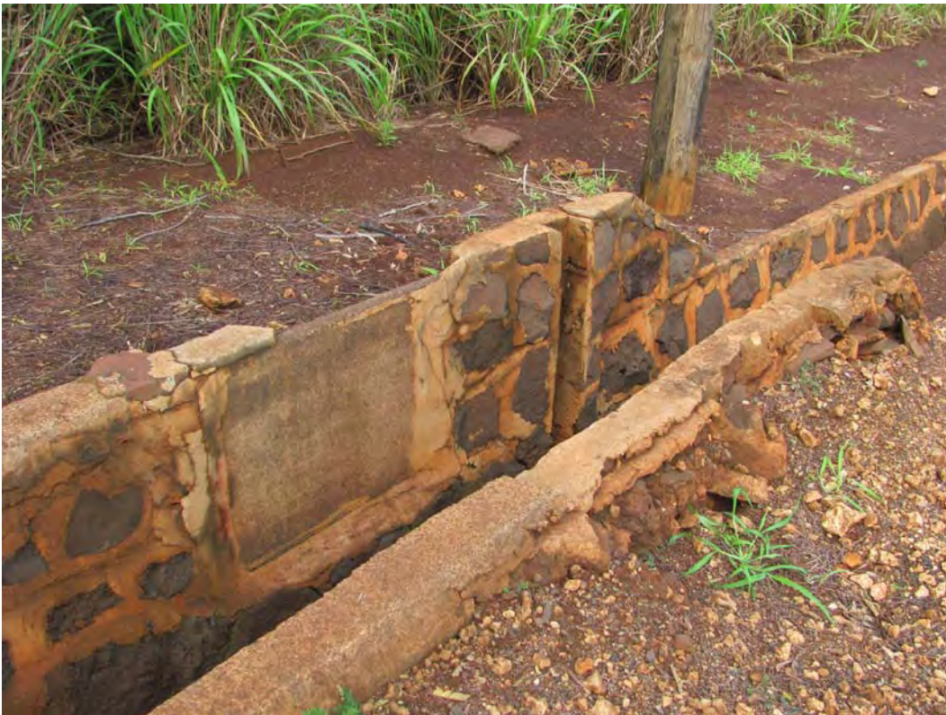
Figure 51. Site 7159 Section 2 third sluice gate complex, view to the south.
