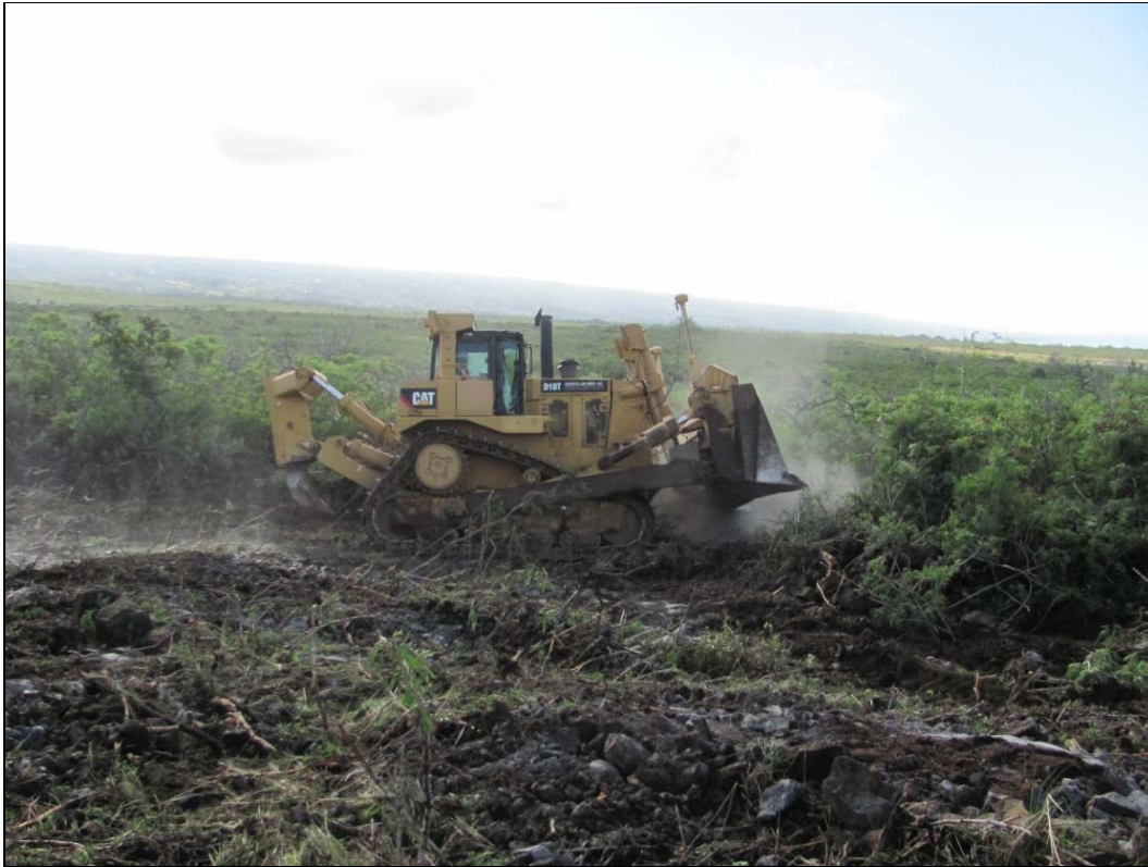
Figure 4. Initial grubbing of the development area with Cat D10T, view to the southeast.
