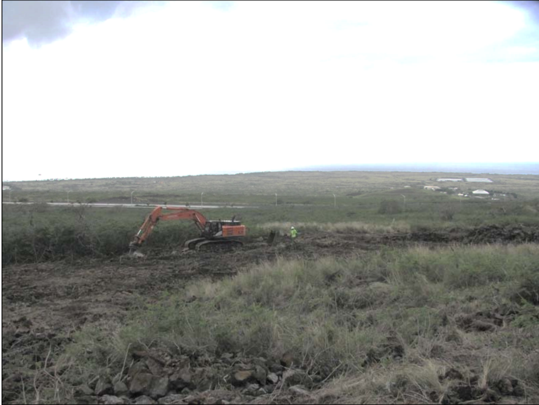
Figure 5. Hitachi 470 LC excavating, view to the southwest.
