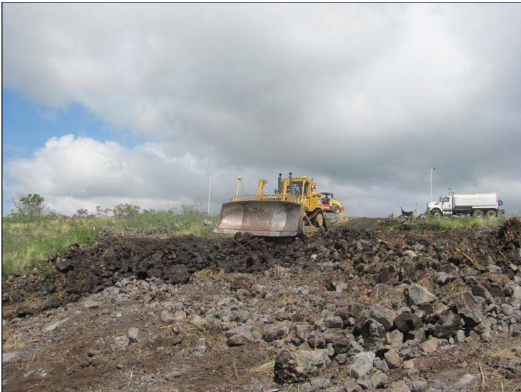
Figure 6. Cat D10T grading, view to the north.
