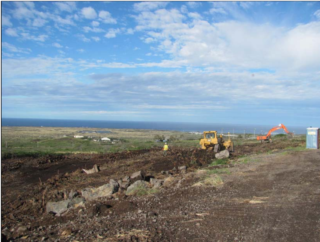
Figure 8. Cat D10T bulldozer and Hitachi 470 excavator working in tandem, view to the southwest.
