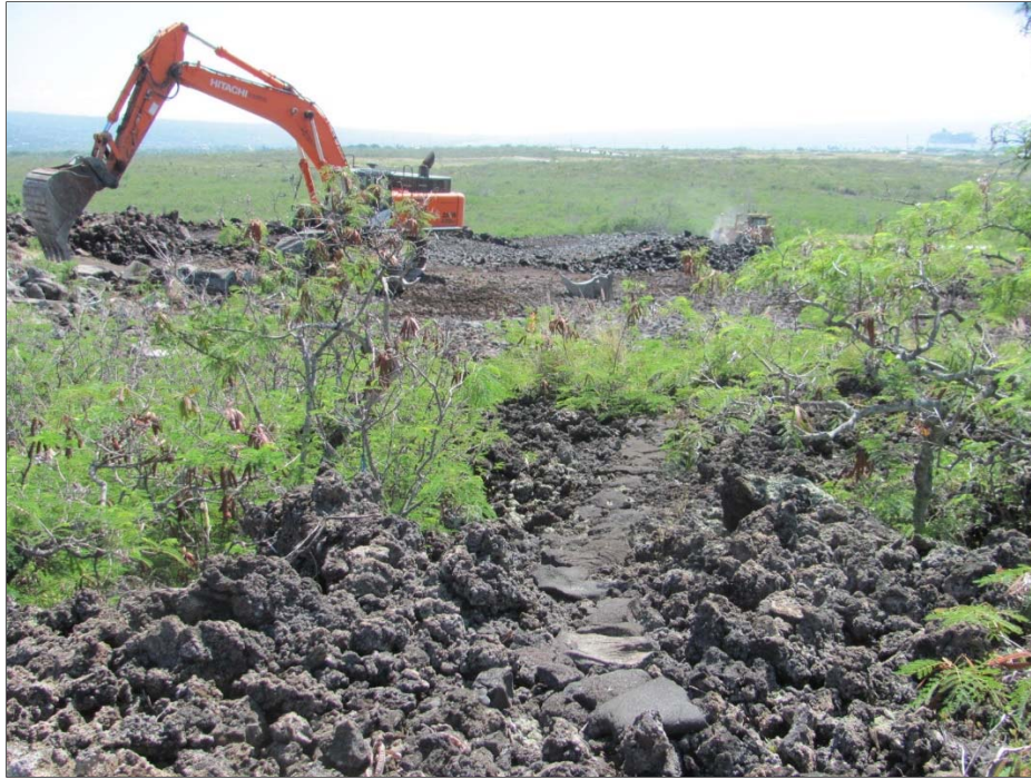
Figure 10. Retained portion of SIHP Site 13207 Feature A, view to the south.
